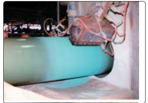
Application of topcoat 3M™ Scotchkote™ 207R to pipe. 9
