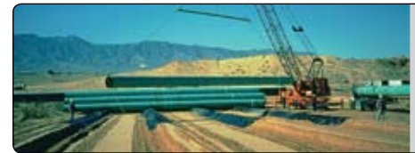
5 Stacked pipe with 3M™ Scotchkote™ coating ready for installation.
