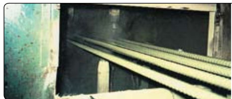
4 Application of 3M™ Scotchkote™ epoxy coating on rebar.
