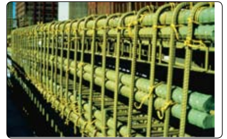
Rebar coated with 3M™ Scotchkote™ 413. 17
