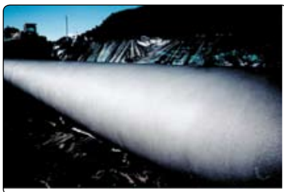
Cleaning pipe to a white finish for a rehab project. 20
