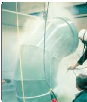
Fluid bed dip application of 3M™ Scotchkote™ 206N.
