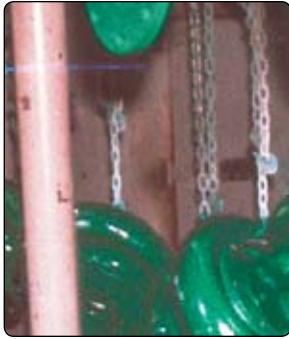
Pump volutes protected against corrosion with 3M™ Scotchkote™ 134.
