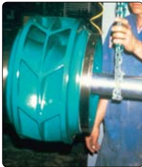
Application of 3M™ Scotchkote™ 134 custom coating on a turbine.
