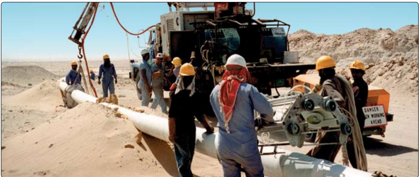
Pipe coated with 3M™ Scotchkote™ Fusion Bonded Epoxy as the primary layer, polypropylene copolymer adhesive and polypropylene overcoating.
