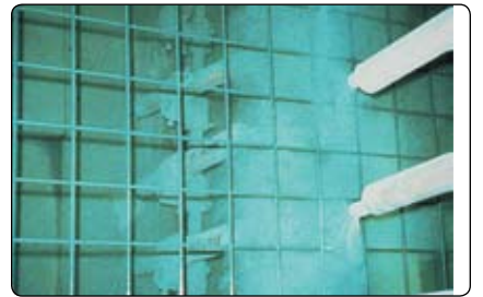
3M™ Scotchkote™ 413 spray grade being applied to wire mesh. 18
