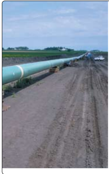
The Alliance Pipeline in Minnesota, coated with 3M™ Scotchkote™ 6233. 7
