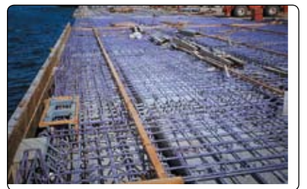
3M™ Scotchkote™ 426 coated rebar in naval pier prior to concrete pour. 19
